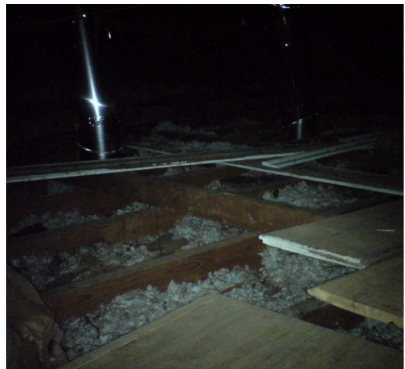
adding insulation and filling in existing voids
