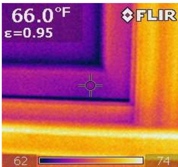
Photos of window air leakage
